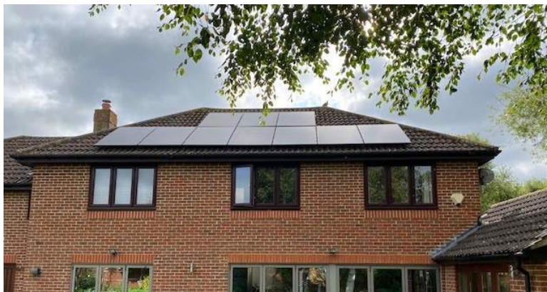
West – 10x395W panels with optimisers
