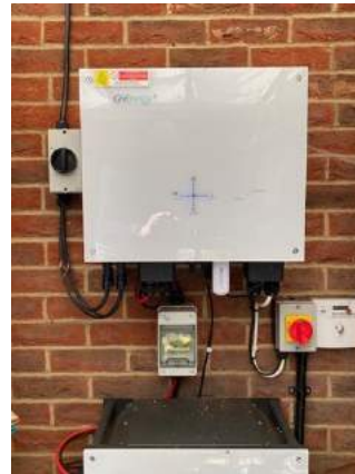
GivEnergy 5kW Inverter
