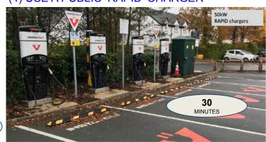
CHARGING TIMES SHOWN HERE ARE FOR A TYPICAL "100 MILE TOP UP" (25kWh)
